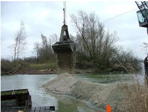
Figure 2: Construction of dams at “Het Groene Eiland”
