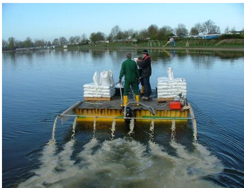
Figure 3: applying a Phoslock ® slurry from a pontoon at “Het Groene Eiland”
